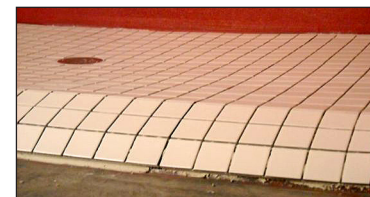
Handi-Kirb with tile installed
